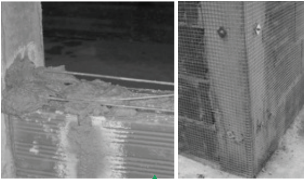
Bed joint reinforcement | Reinforced plaster
