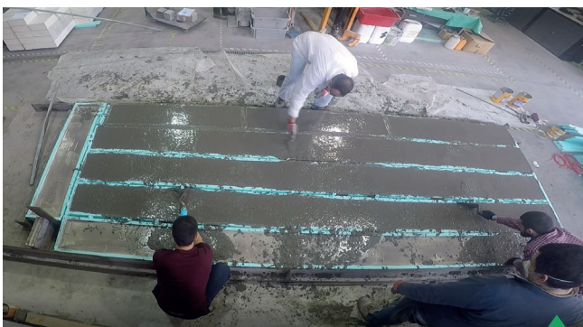
Casting the top FRC layer
