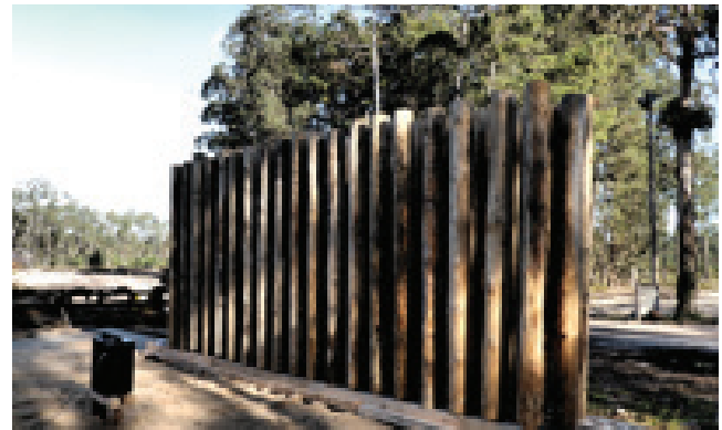
Image of the timber log assembled structure.
