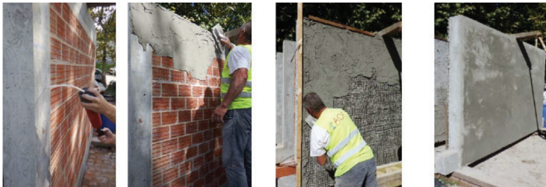
Strengthening of masonry infills
