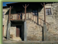
Trás-os-Montes Schist construction.
