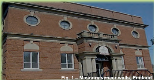
Fig. 1 – Masonry veneer walls, England
