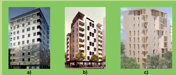
Fig. 1 - Constructed buildings using CLT. a) Stadthaus, London (9storeys); b) Forté, Australia (10 storeys); c) Via Cenni, Milan (10 storeys)
