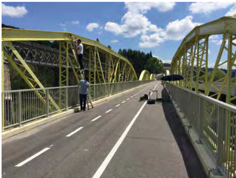
Fig. 2 Portela Bridge in Coimbra
