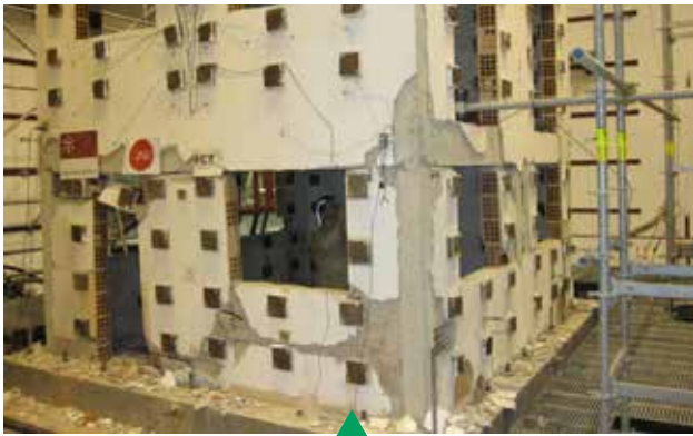
Model 2 north and west elevation after shaking table test.
