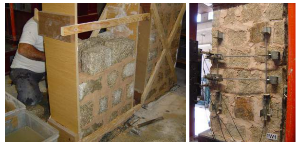
Figure 2 – Construction and testing of the first series of multi-leaf masonry walls.
