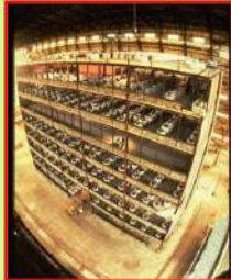
Steel building - Cardington
