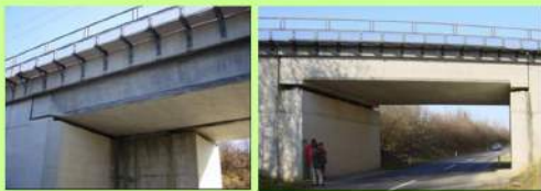
Abutments of a twin slabs viaduct
