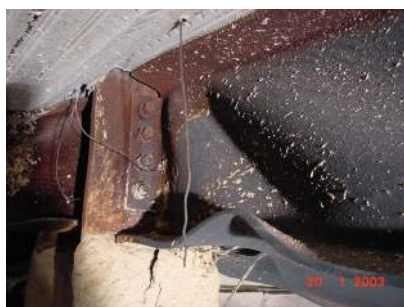
Fig. 5 – Local Buckling.
