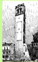
Fatigue collapse of Pavia Tower, 1989, Italy
