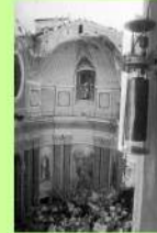
Fatigue collapse of Noto church, 1996, Italy
