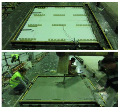
Fig. 5 Casting of sandwich panels.
