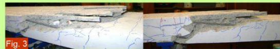
Failure of the strengthened slab strip by the detachment of the strengthened concrete cover layer or due to the formation of a shear failure - hogging region.
