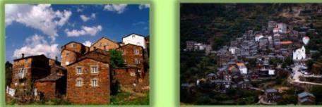
Schist masonry constructions.
