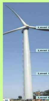
Wind tower instrumentation levels
