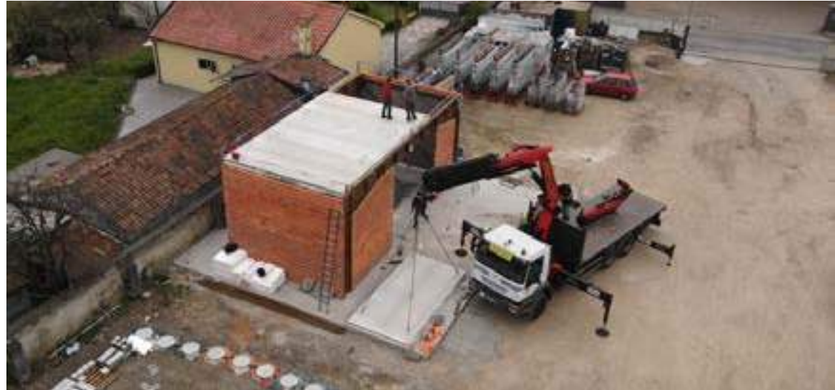
Building a real scale facility with a pavement made by PreSlabTec slab modules.
